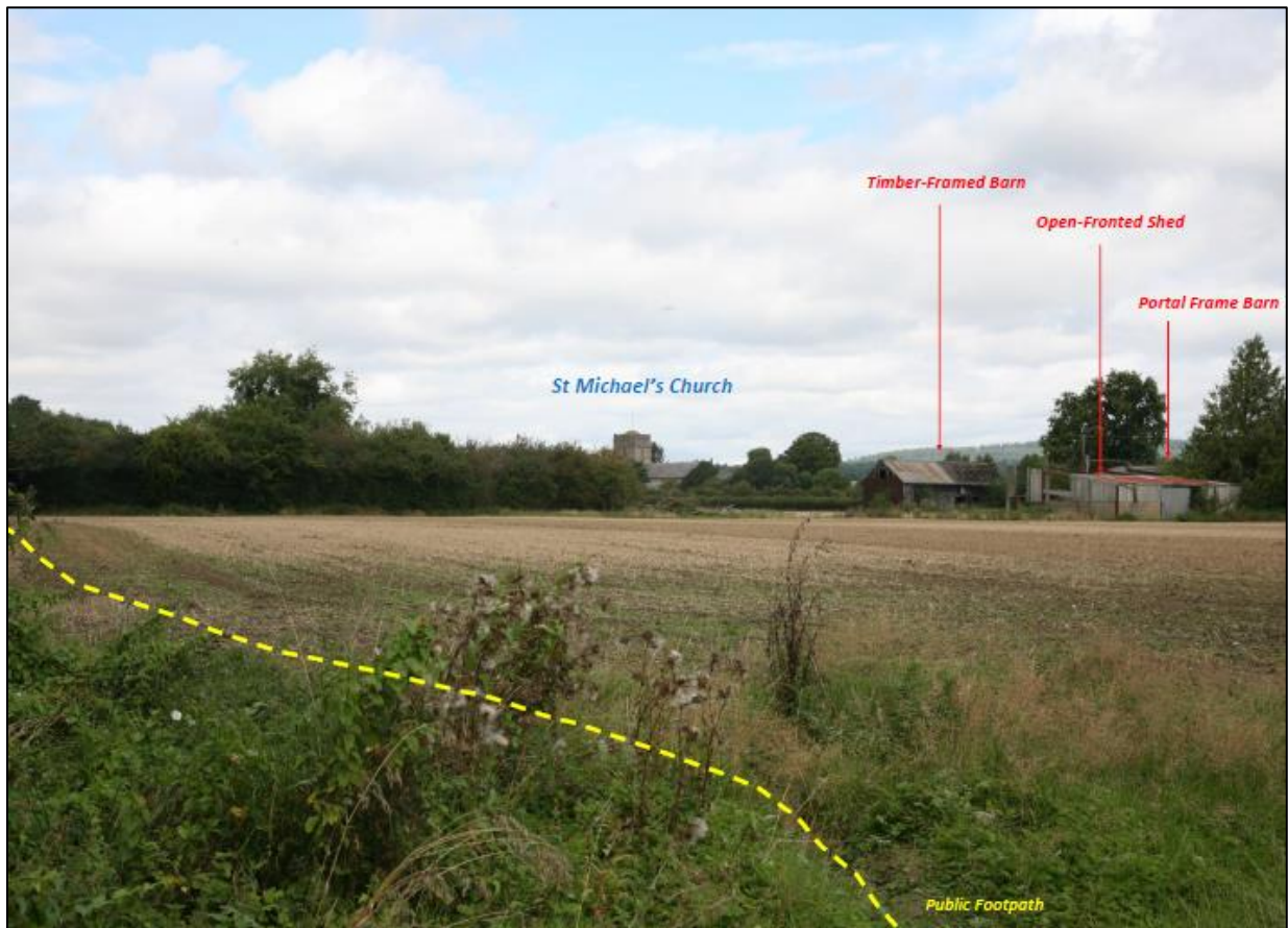
Figure 4: View from footpath KL3 looking north west
